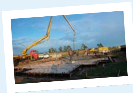
Pictured above: Construction in progress
